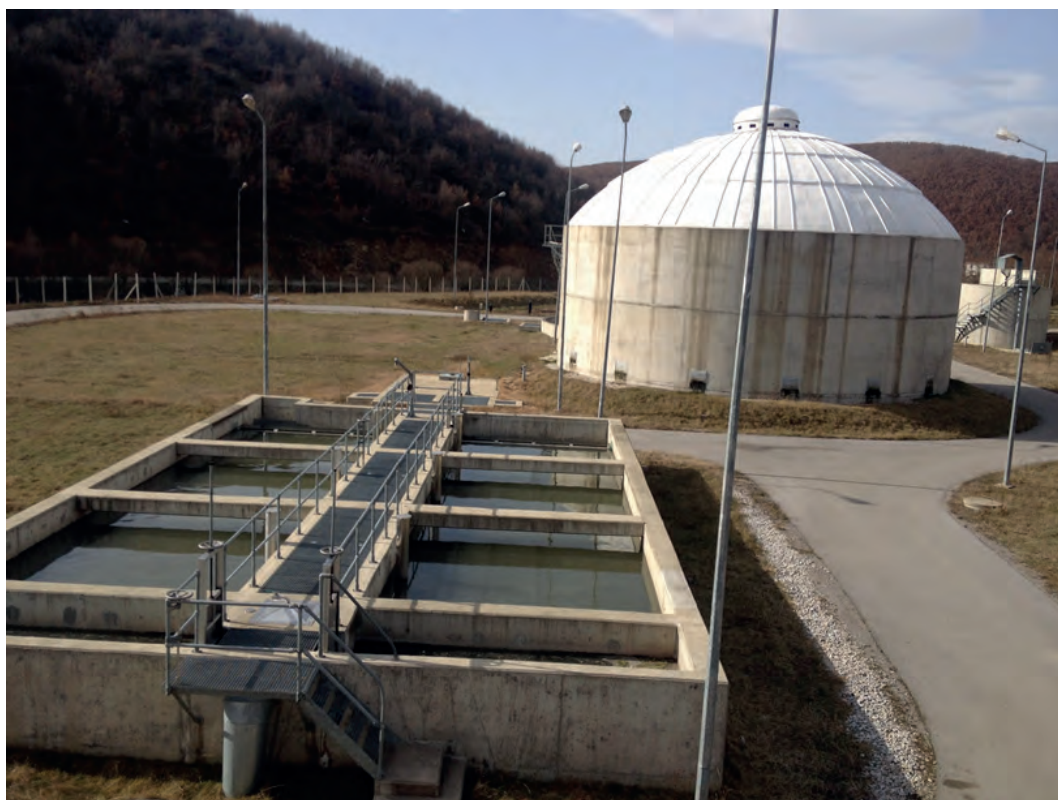
Figure.52. Wastewater Treatment Plant in Skenderaj
