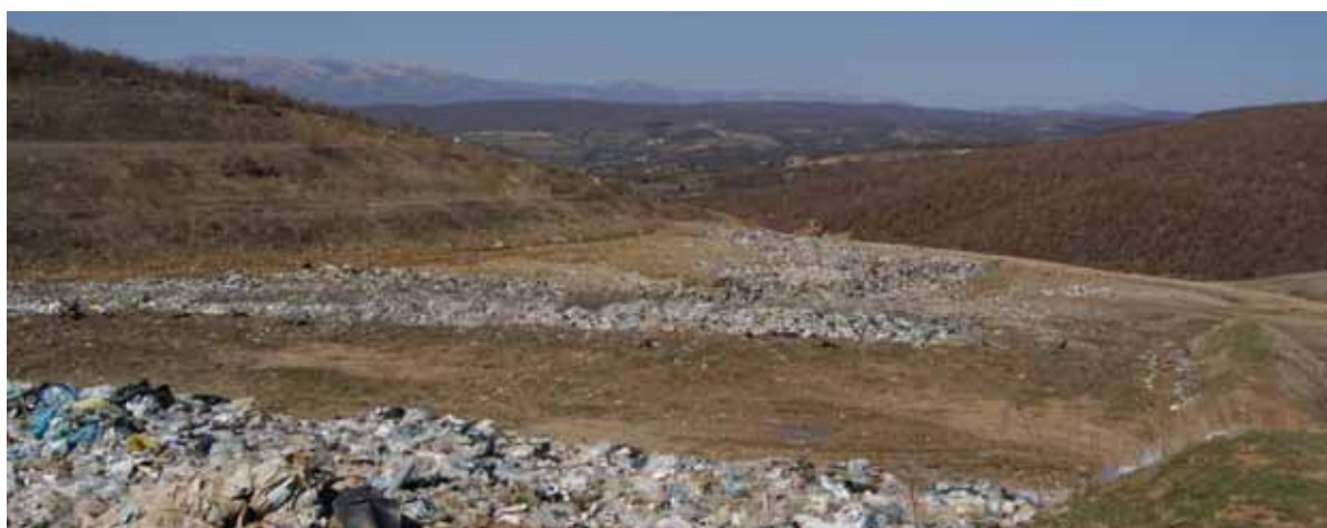
Sanitary landfill in Podujevë
