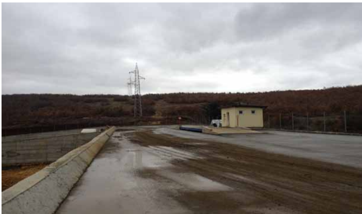
Waste transfer station in Drenas
