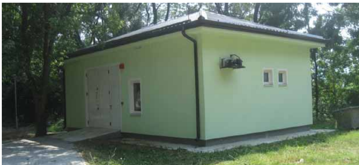
Medical waste treatment plant in Gjakovë
