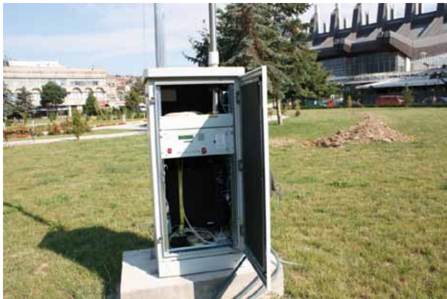
Air quality monitoring station located at ex Rilindja yard.
