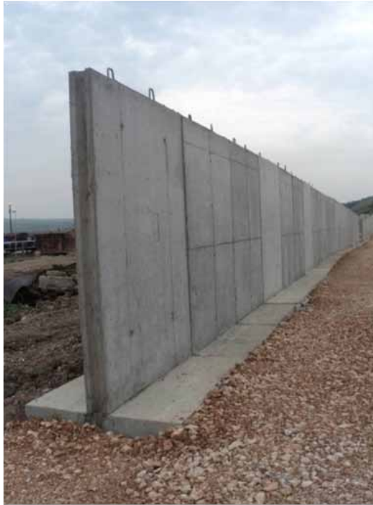
A view of noise barrier (concrete wall) in Sibofc
