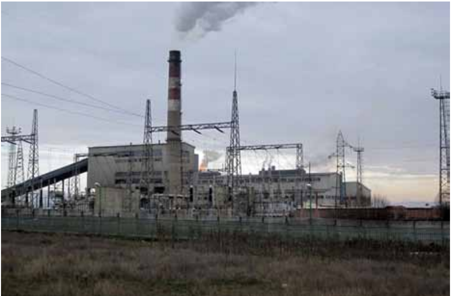
The Ferronikeli complex in Drenas
