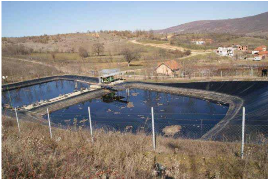
Waste water collected at the sanitary landfill in Gjilan
