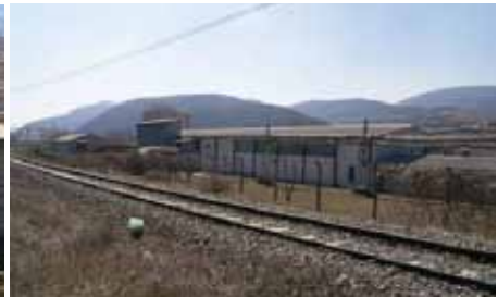
Factory for production of Salonite
