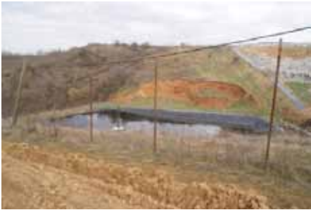
Accumulated waters at the landfill
