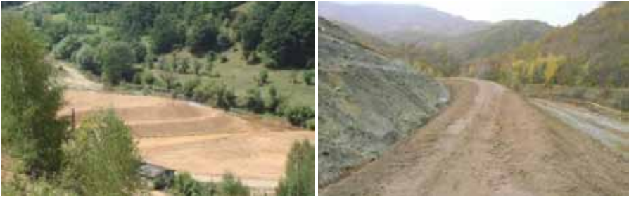
Rehabilitation of Artana tailings 11
