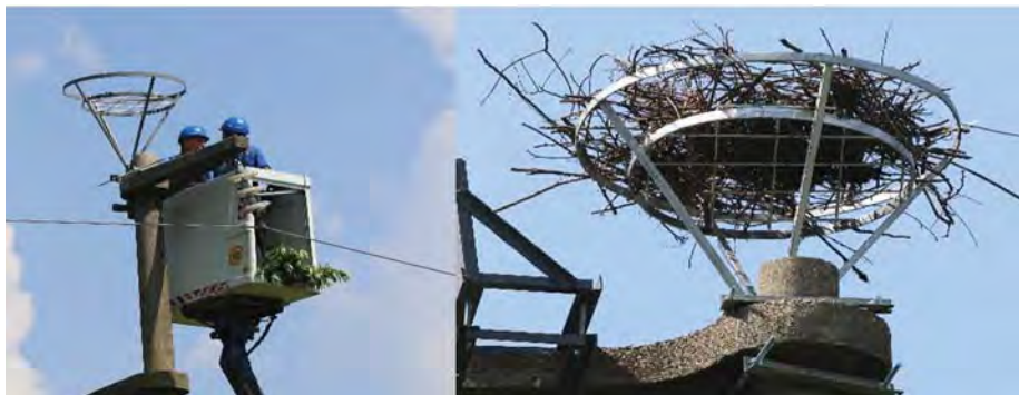
Image No. 123. Installing a platform for stork nests
